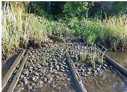
The author took this photograph (above) of the brick ferry landing July 11, 2016. Bricks and wooden beams re-enforced the docking port. The landing and main avenue to Dean Hall were visible from the ferry dock.
